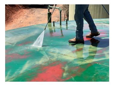
Pressure washing in process- SSPC-SP WJ-4 Light Cleaning
