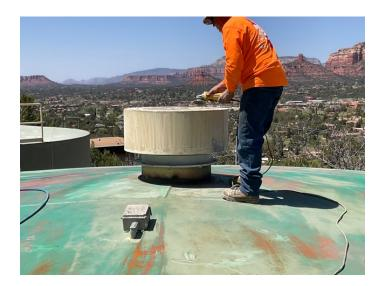
Surface preparation in process- SSPC-SP3 Power Tool Cleaning (grinder)
