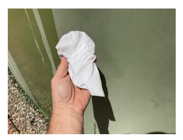
Clean cloth used to verify removal of chalking and contaminates. Surface cleanliness acceptable.
